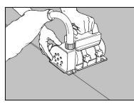
The joints are chamfered or grooved to about 2/3 of the thickness using a hand grooving tool or machine prior to welding. Never reach the foam backing when existing.
